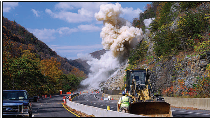
Rock blasting in an effort to clear and stabilize the slide.
